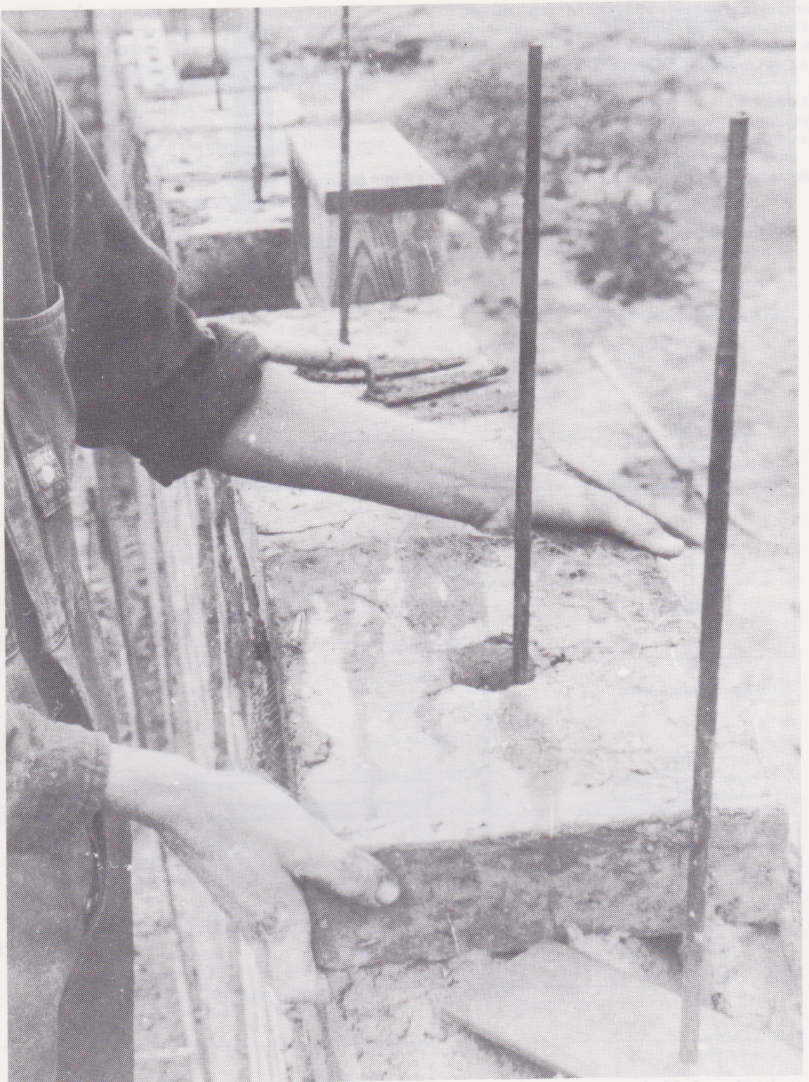
Fig. 1.5 – Top plate holding-down bolts being built into an adobe wall
