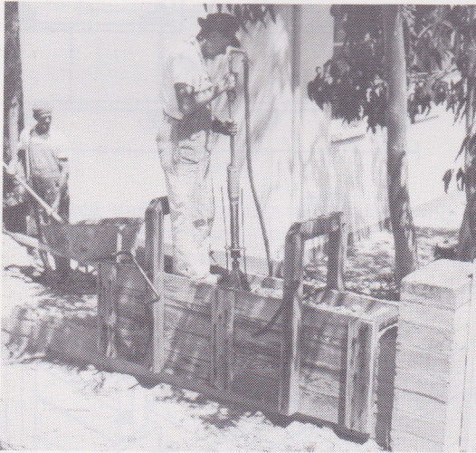
(b) Roller-supported formwork
