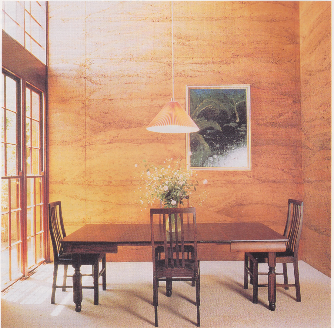
Fig. 4.7 – Interior wall of rammed earth Photo Courtesy Ramtec Pty. Ltd.
