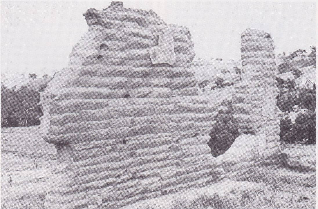
Fig. 4.3 – Different erosion of the top and bottom of layers of rammed earth
