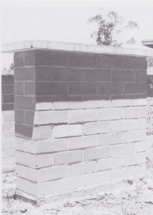
Fig. 6.8 – Demonstration walls built of Cinva-ram on the NBTC grounds.
