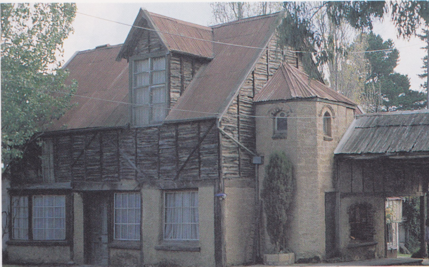
Fig. 3.2 – A section of 'Montsalvat', built of adobe about 1940
