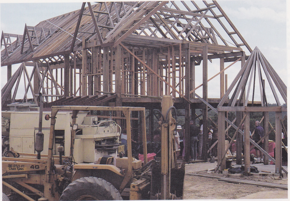
Fig. 1.10 – Sawn-timber framed house under construction
