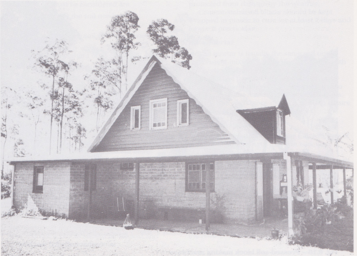
Fig. 6.7 – A house built of Cinva-ram type blocks
