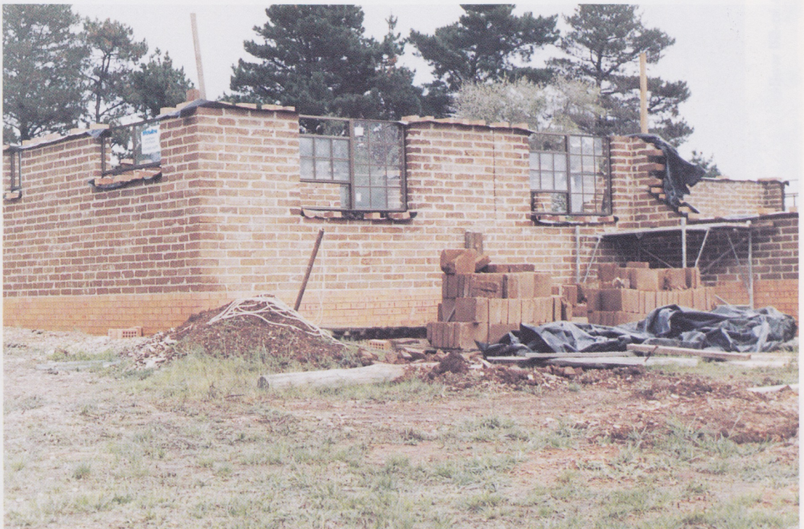
Fig. 6.11 – House incorporating pressed-soil blocks under construction
