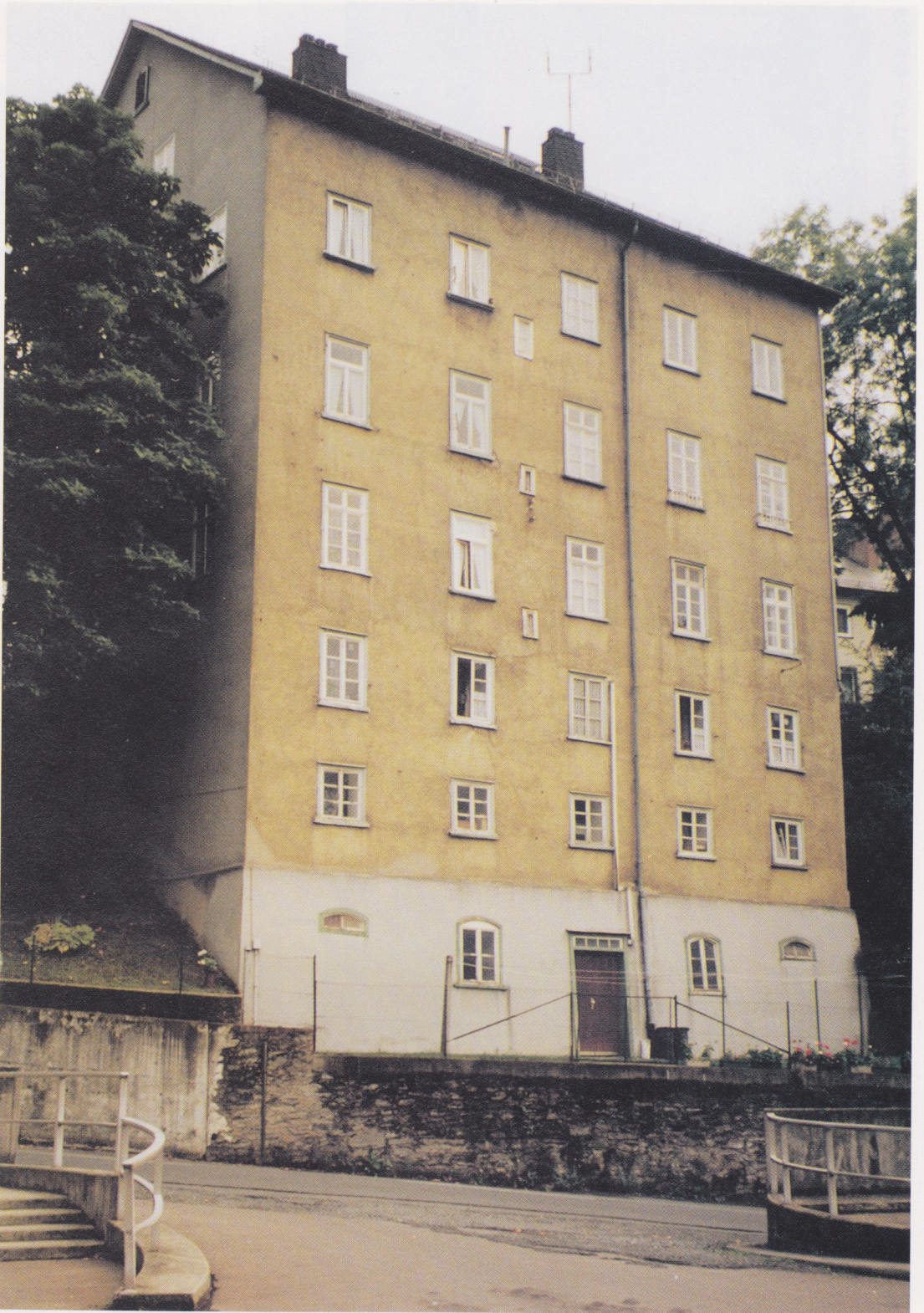
Fig. 4.10 – A six storey loadbearing rammed-earth building at Weilburg, F.G.R. constructed in 1826
