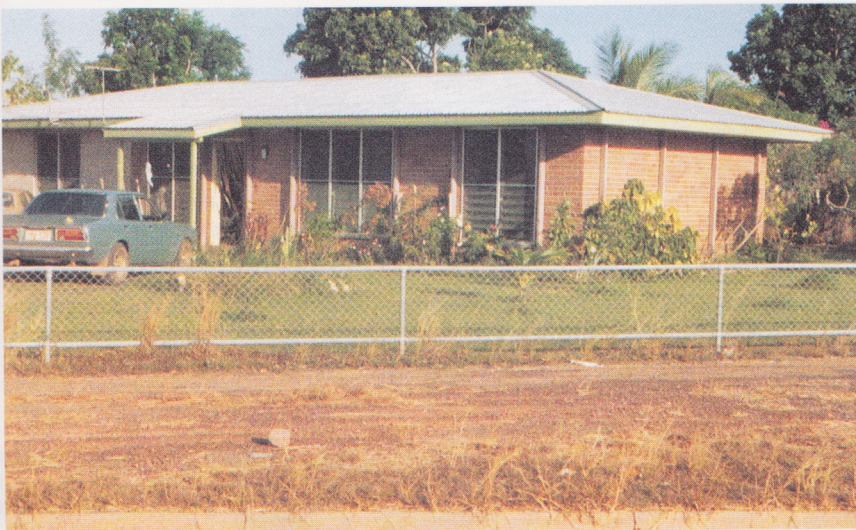
Fig. 3.3 – A typical house built by the Northern Territory Housing Commission from stabilised- earth bricks
