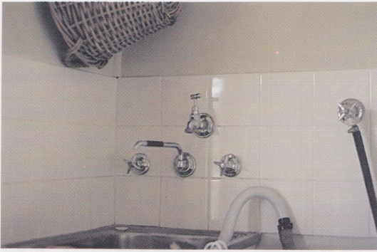
Fig. 1.8 – Wet area showing render and tiling
