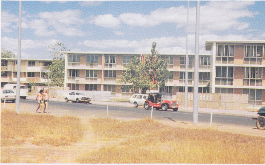
Fig. 3.4 – A block of flats in Darwin built of stabilised-earth bricks by the Northern Territory Housing Commission
