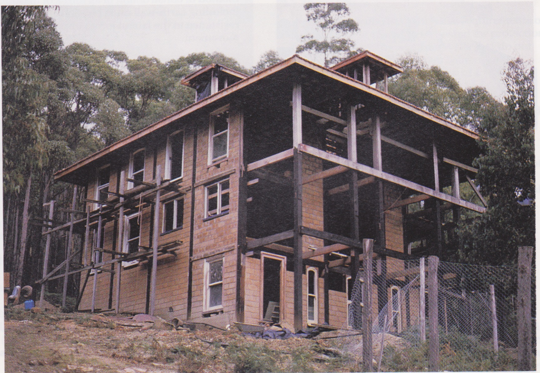
Fig. 1.11 – Sawn-timber framed house under construction
