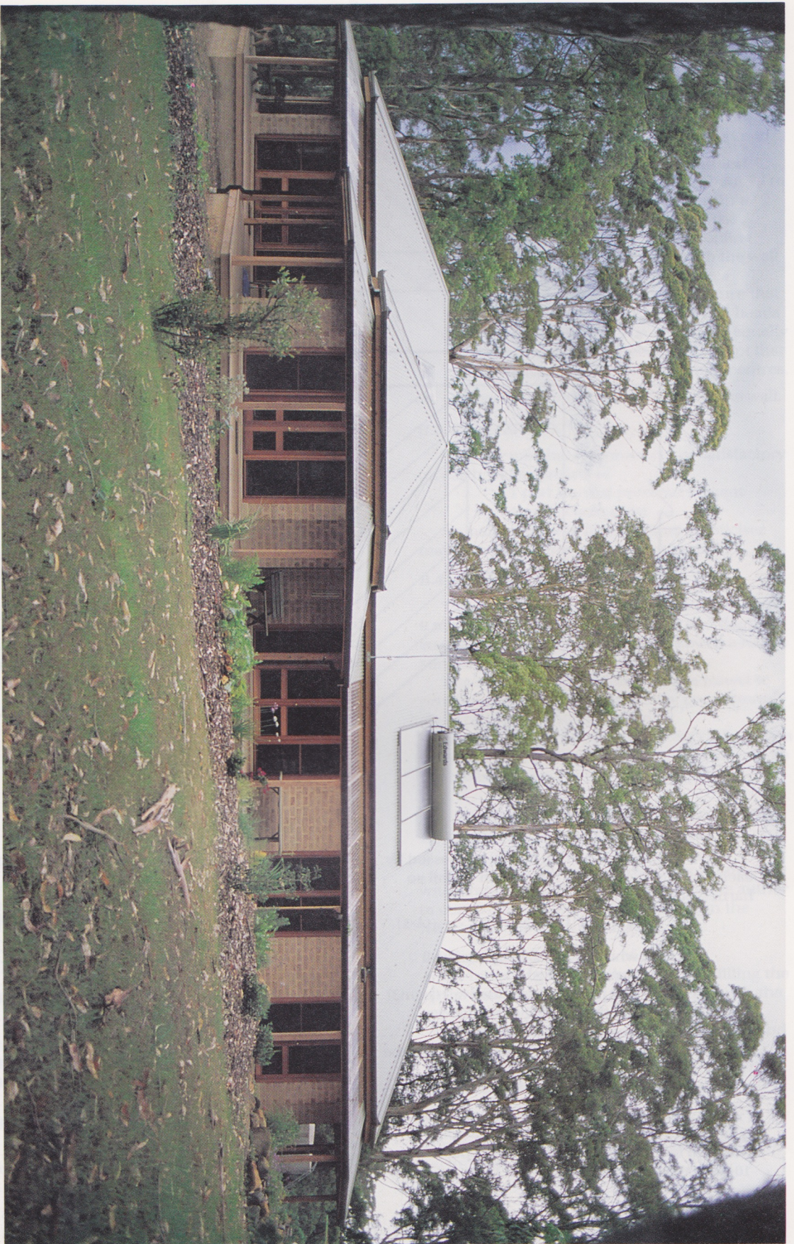
Fig. 6.13 – House with load-bearing cement-stabilised pressed-soil block walls
