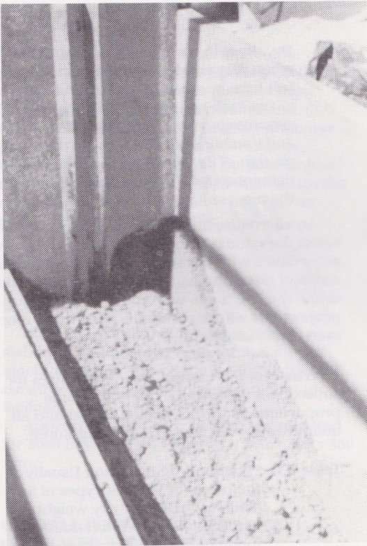
(a) render mix and core soil as placed in forms
