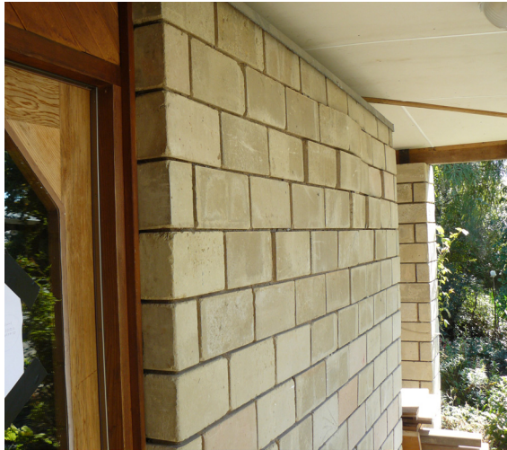
Figure 20 Burwood single storey post and beam house with pressed brick walls showing upper level damage
