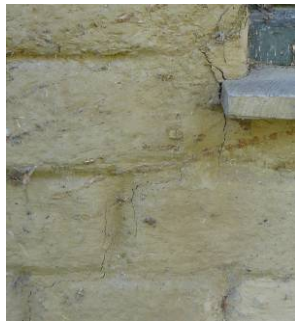
Figure 14 Typical cracks adjacent to window
