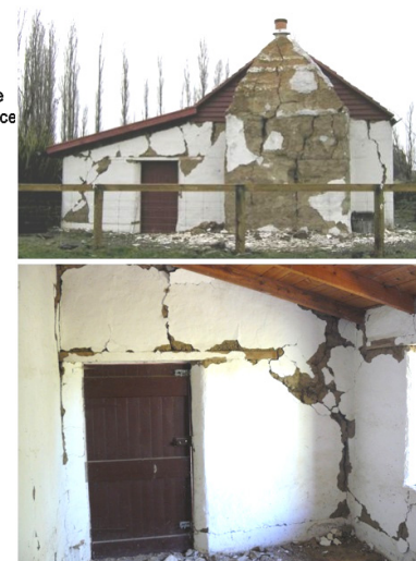
Figure 2 Cotons cob cottage extensively damaged
