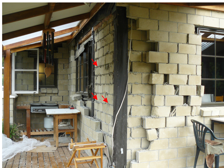
Figure 19 Little River post and beam house with pressed brick infill walls. Lower storey shows a post and damaged exterior double skin cavity walls with some remaining pulled out ties between wythes indicated.
