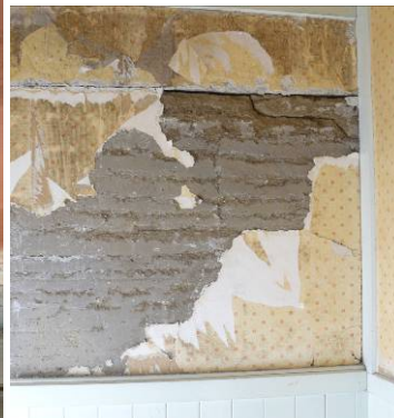
Figure 6 Hororata house showing offset of the bond beam outside and inside and a related wall crack
