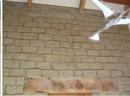
Figure 15 High wall above lintel (vertical crack not visible)
