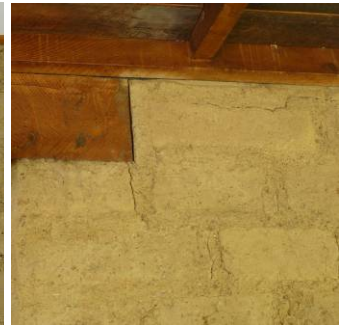
Figure 11 Opening at edge of lintel beam
