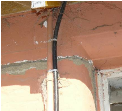
Figure 6 Hororata house showing offset of the bond beam outside and inside and a related wall crack
