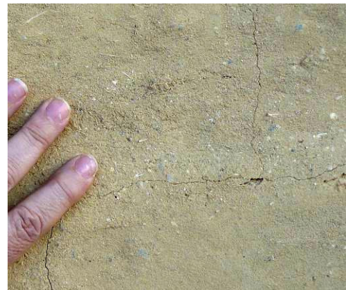
Figure 18 Cracking through plaster showing fractures at mortar joints
