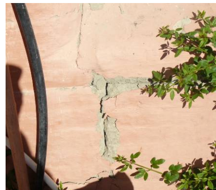
Figure 6 Hororata house showing offset of the bond beam outside and inside and a related wall crack
