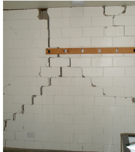
Figure 21 Burwood house internal infill double skin cavity wall showing major damage.
