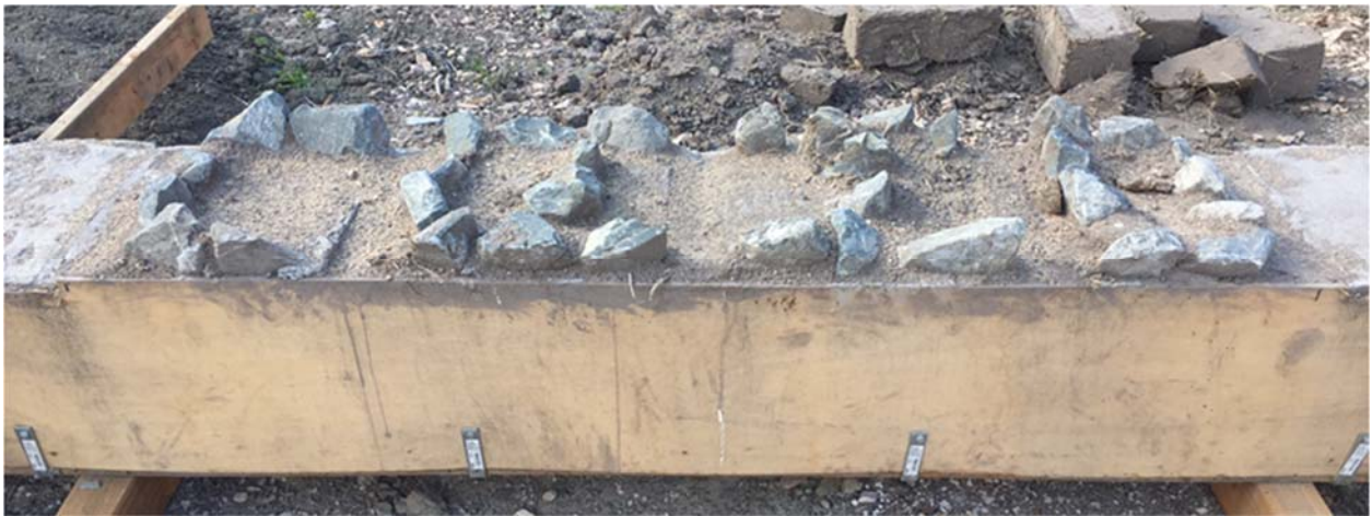
Figure 3: Wall 1 Base Design (Common Practice).
