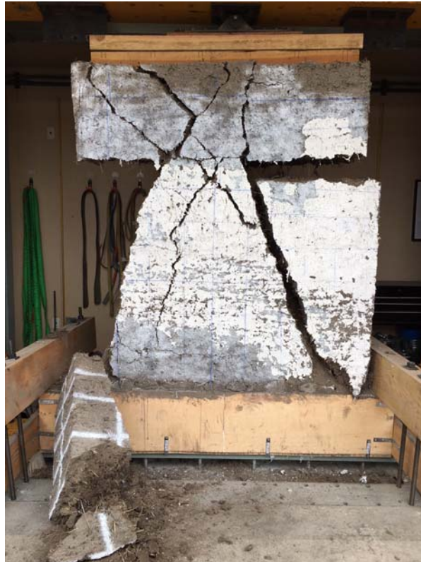
Figure 10: Wall 1 (Common Practice) After Testing.
