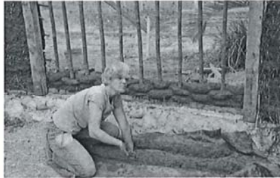
Fig 11. "snake-like" cobbing method around wattle frame
