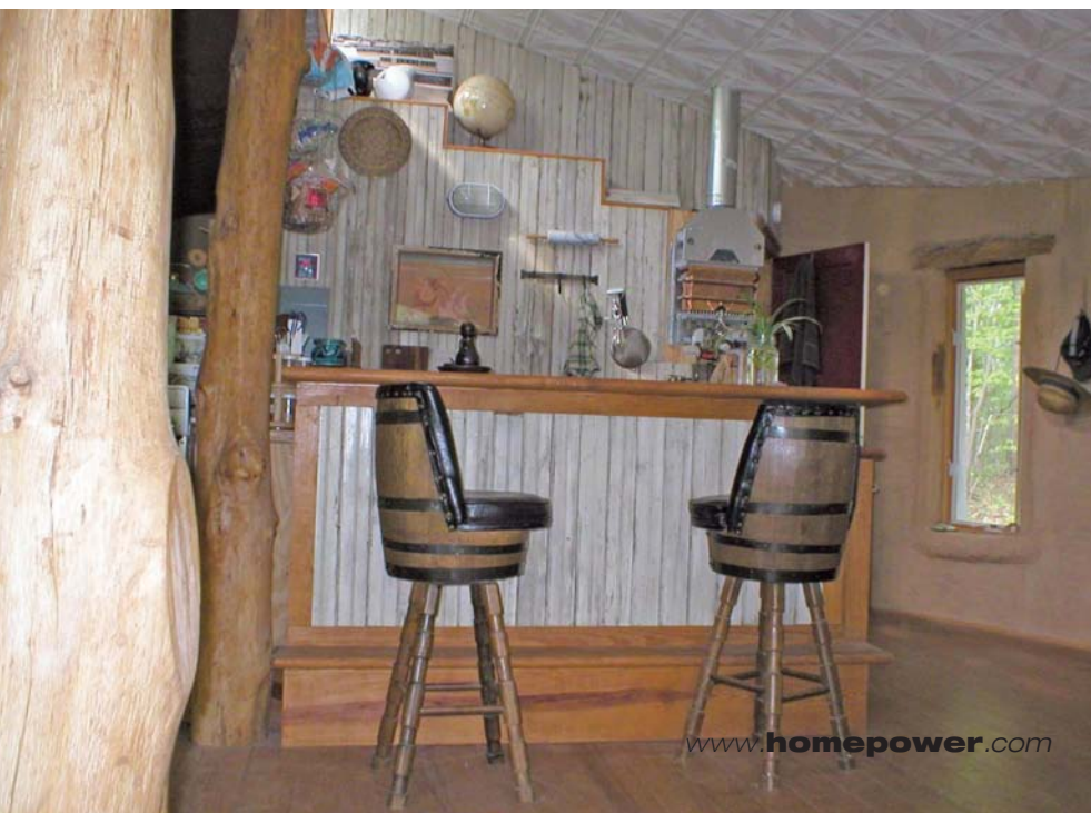
Additional support in the center of the house was necessary to transfer a portion of the roof's load directly to the ground rather than to the walls.
