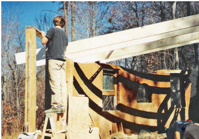
The author places the first rafters in the cob walls, after “keying” them to lock them into place.
