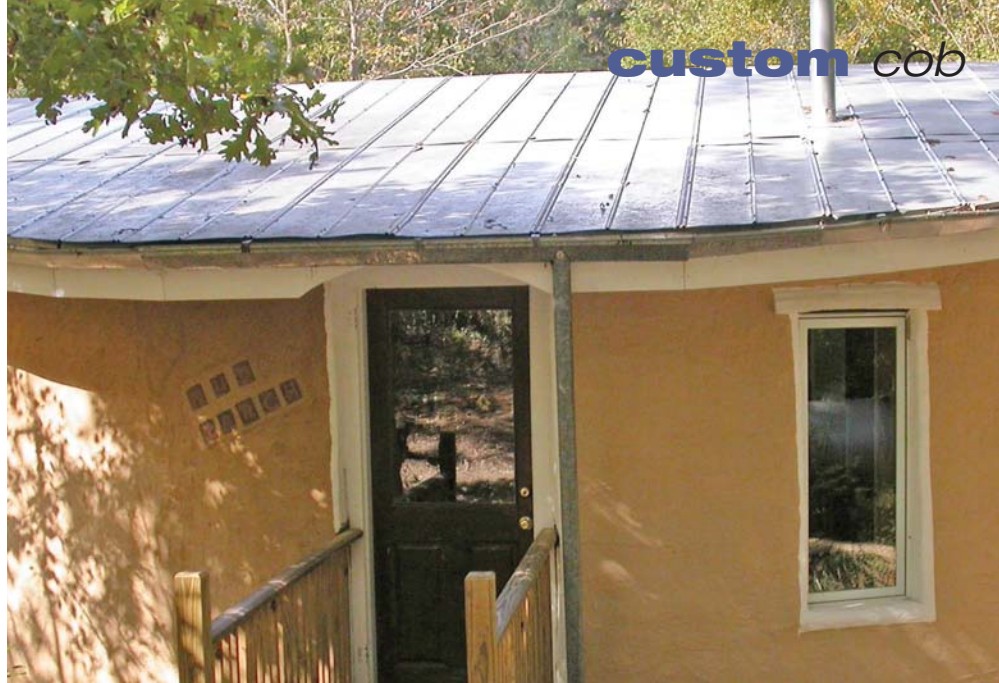
This gently sloped roof puts less weight on the cob walls while simultaneously providing enough of an angle to shed snow.
